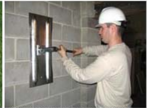
Step 6: Anchors can be tightened at intervals and straighten the wall over time.
