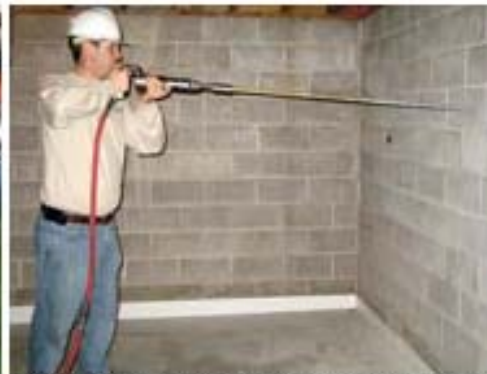
Step 2: A small hole is drilled through the wall and a rod is driven out.
