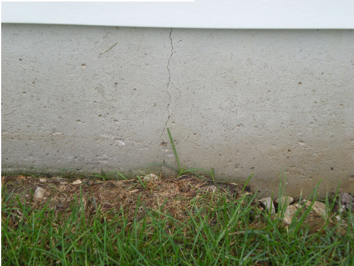
现浇混凝土墙 纵向裂缝 (Vertical crack in cast in place concrete wall)
