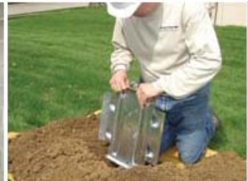
Step 3: An earth anchor is installed and attached to the rod.
