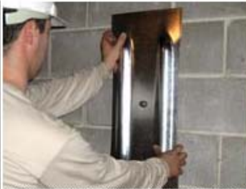
Step 4: A wall plate is attached and tightened, sealing the earth anchor.
