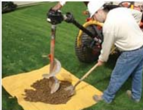
Step 1: Sod is carefully removed and an earth anchor hole is augured.
